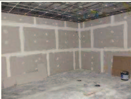
Execu??o paredes dry wall
