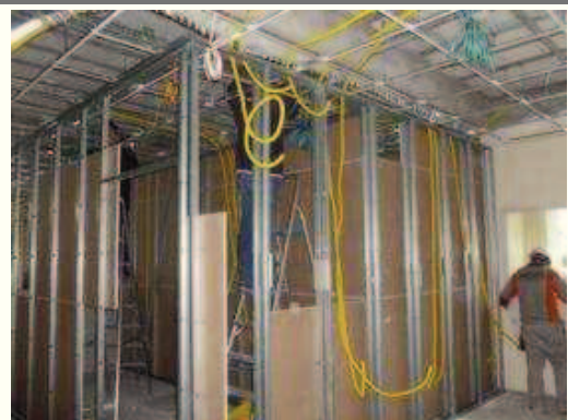
paredes Dry Wall
